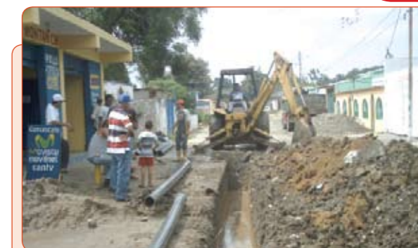
Installation of 2,000 feet of a 4" polyvinyl chloride pipe
