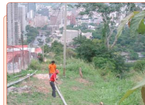
Volunteers move the pipes
